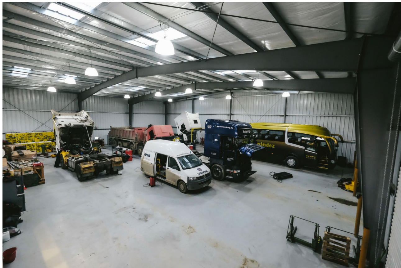
Metal Building Example
