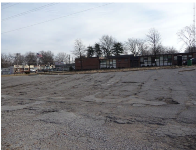
Existing deteriorated asphalt at Bus Stop.
